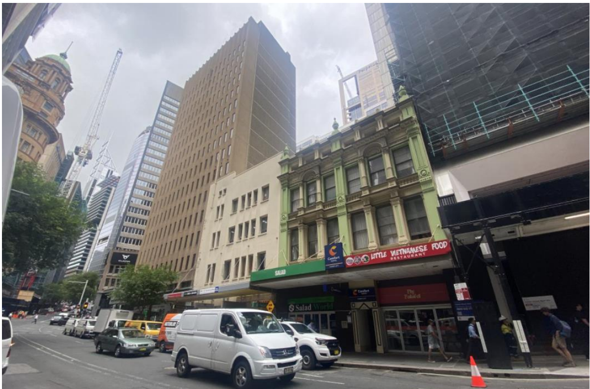
Figure 3: 15-17 Hunter Street, 19-21 Hunter Street and 23 Hunter Street (as viewed from Hunter Street facing south)
